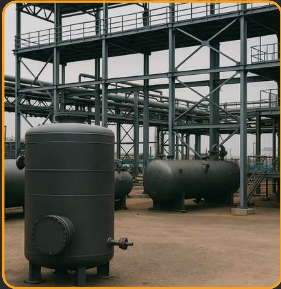
Steel Fabrication & Erection
