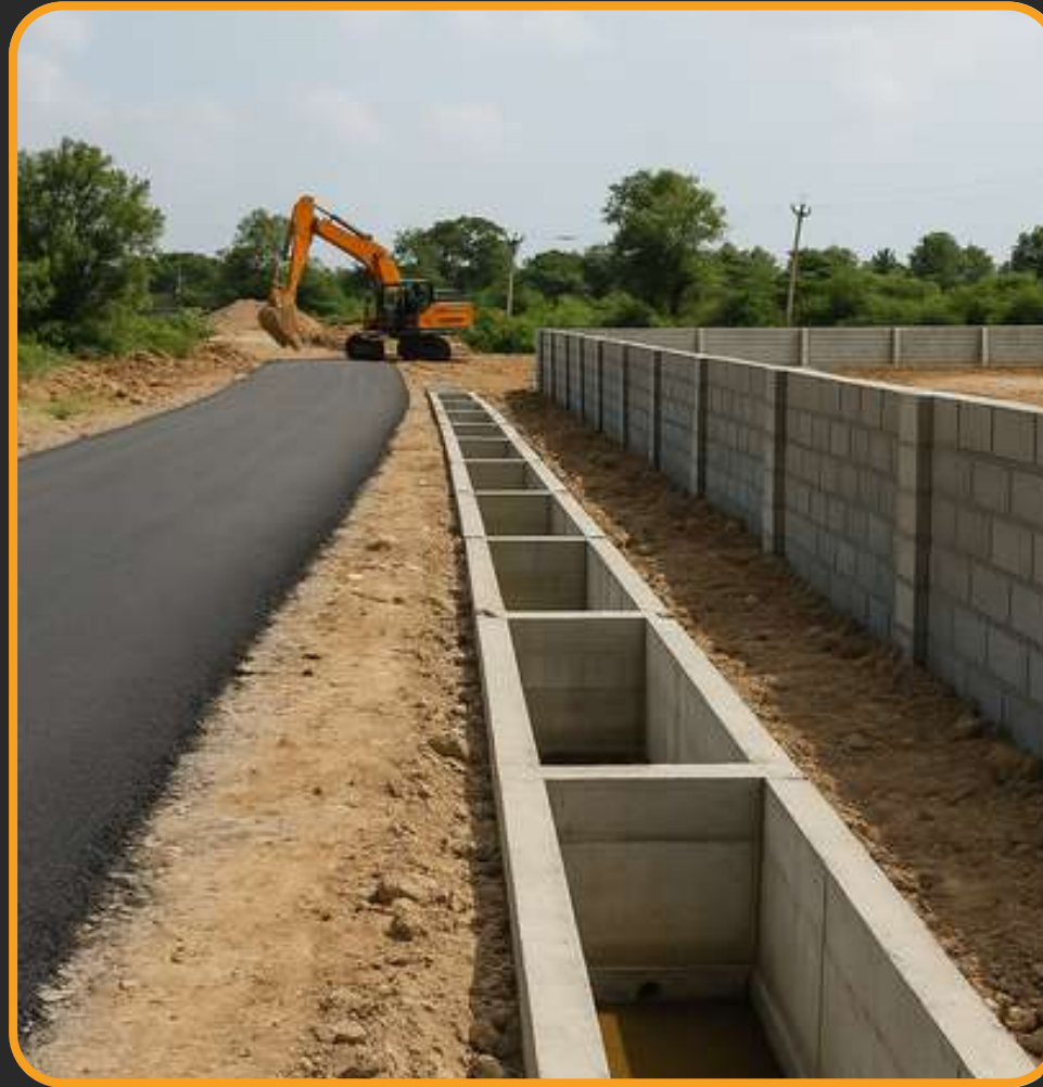
Road & Infrastructure Works
